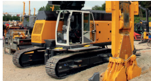
since 2004 CSM Soil mixing Here: Side cutter, 2012
