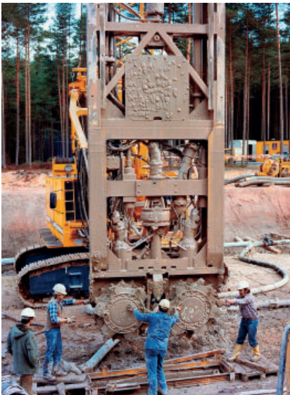
First Bauer cutter 1984 BC 30 cut-off wall at Brombach reservoir
